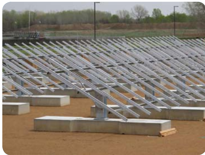
Figure 5: High-density Pre-cast Concrete System (photo: Solar FlexRack)
