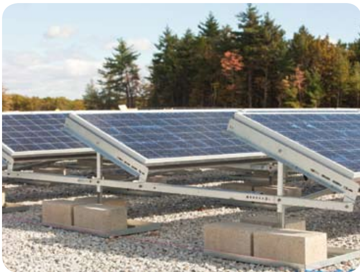
Figure 4: Massachusetts-manufactured Panel Claw Mounting System (photo: Nexamp)
