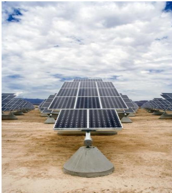
Figure 3-6: 2-MWp PV system with fixed tilt on former landfill in Fort Carson, Colorado
