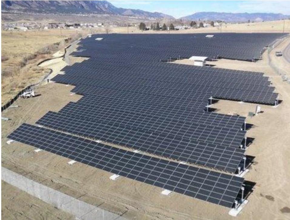
Figure 3-6: 2-MWp PV system with fixed tilt on former landfill in Fort Carson, Colorado
