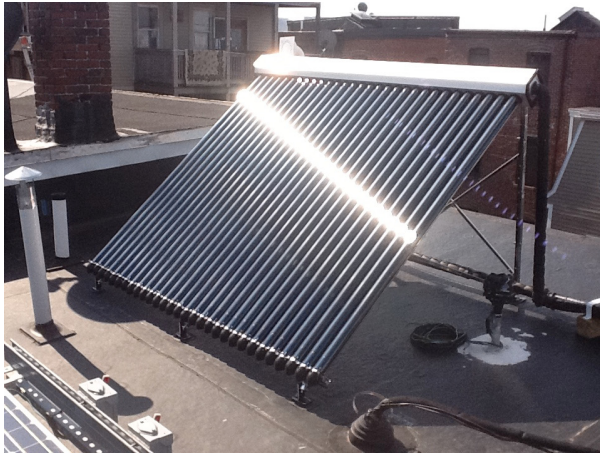
Residential Evacuated Tube System - Boston, MA
