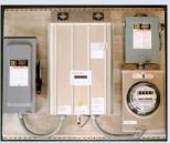
**Inverter** turns DC power to AC power; connects to **meter**, **monitoring system**
