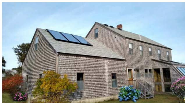
Solar hot water system
