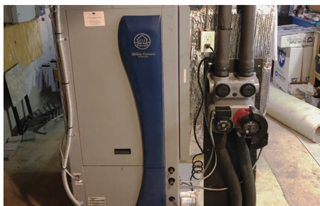
Ground-source heat pump indoor unit
